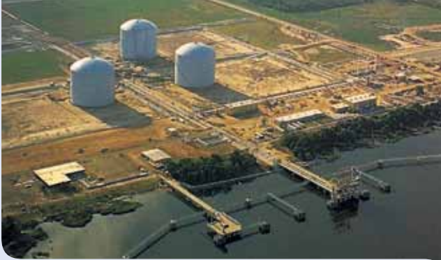
The Elba liquefied natural gas terminal in Georgia near Savannah significantly increased its storage and loading capacities. The $200 million project was completed in July 2010.
