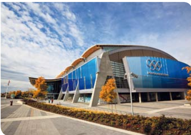
Rexel is involved in a number of infrastructure projects for the Vancouver Winter Olympics - Canada
