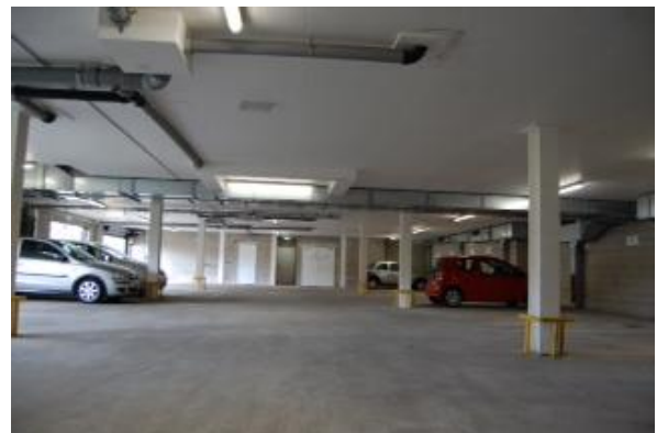
Car park utilised existing fittings with replacement LED tubes
